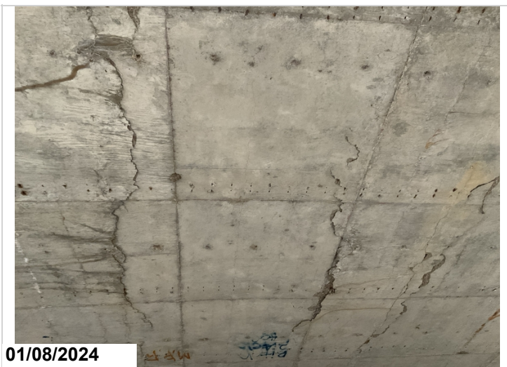
Span #1 soffit-under surface delaminated areas.
