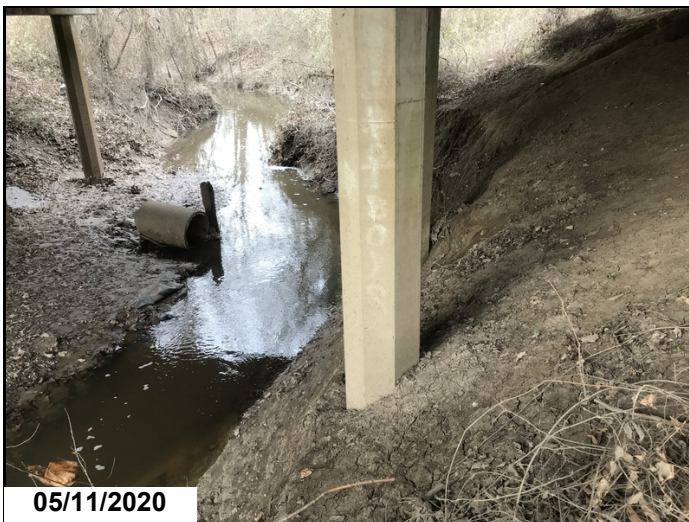
Bent #3 slope erosion.
