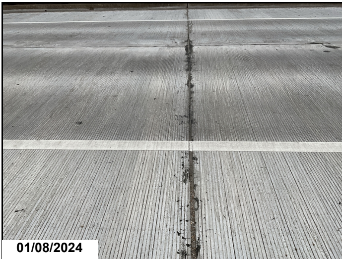
Joints have been replaced since last inspection.
