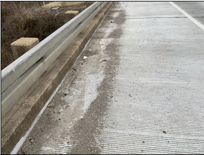
Typical debris in gutters
