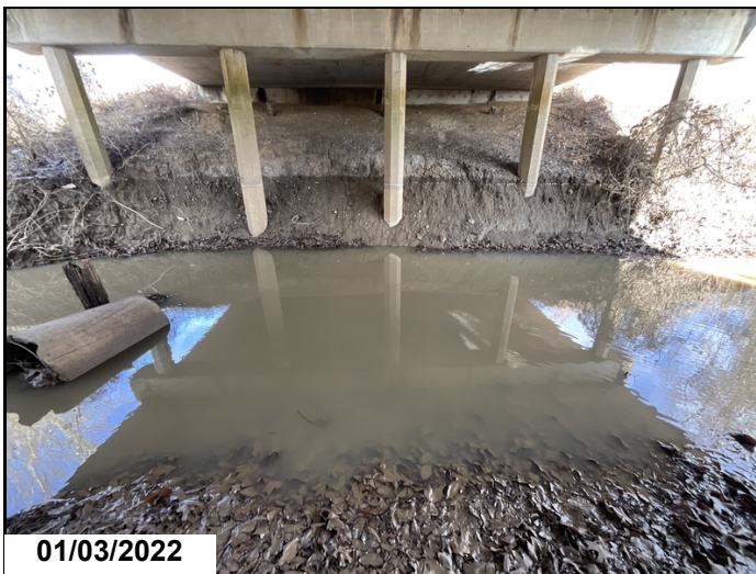
Erosion at bent #3.
