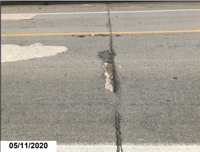
Span #2 has a two foot spall with no exposed rebar in left lane at bent #2.
