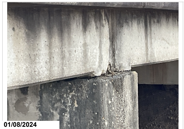
Span #1 slab right side at bent #2 has vertical crack and minor spalling at end of slab
