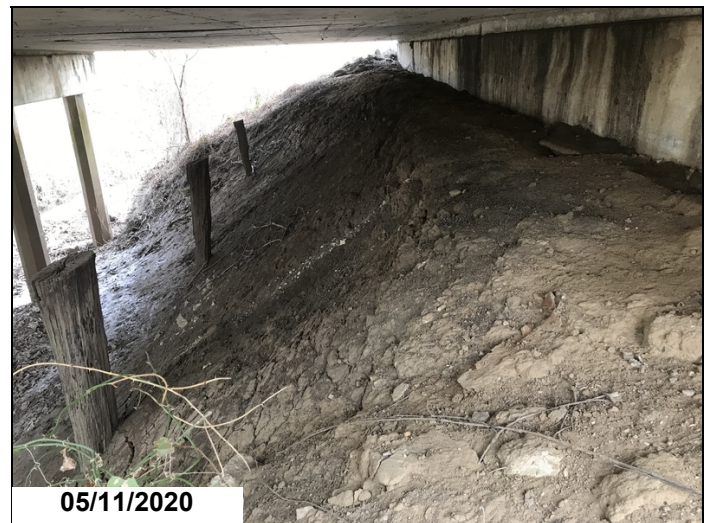
Abutment #1 slope erosion.
