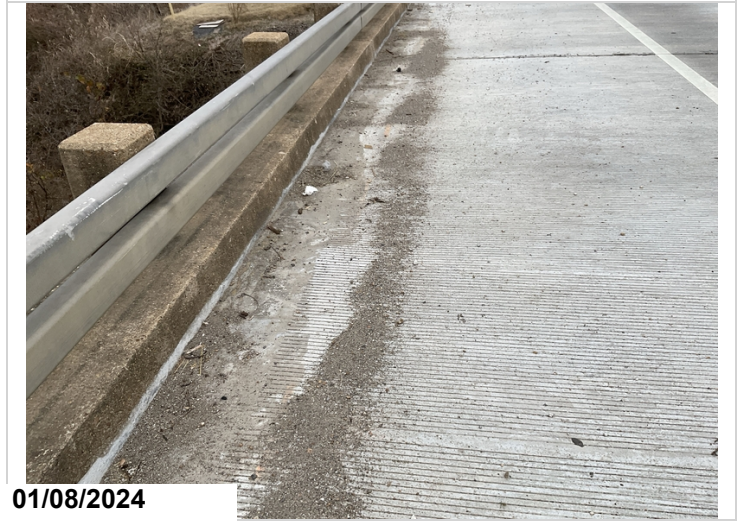
Typical debris in gutters
