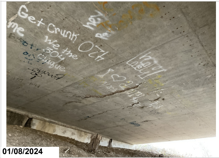
Span #3 soffit-under surface delaminated area
